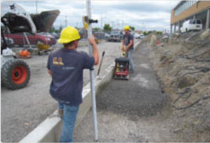
Carefully level and compact the 0-20 mm granular base course.
