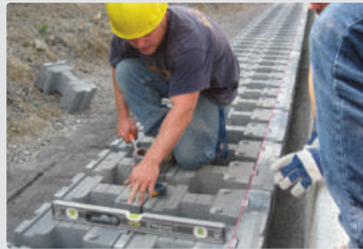
Check the horizontality of the stabilizing blocks installed
