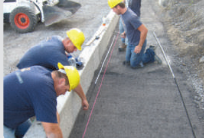
Spread loose granular bedding with a maximum thickness of 20 mm
